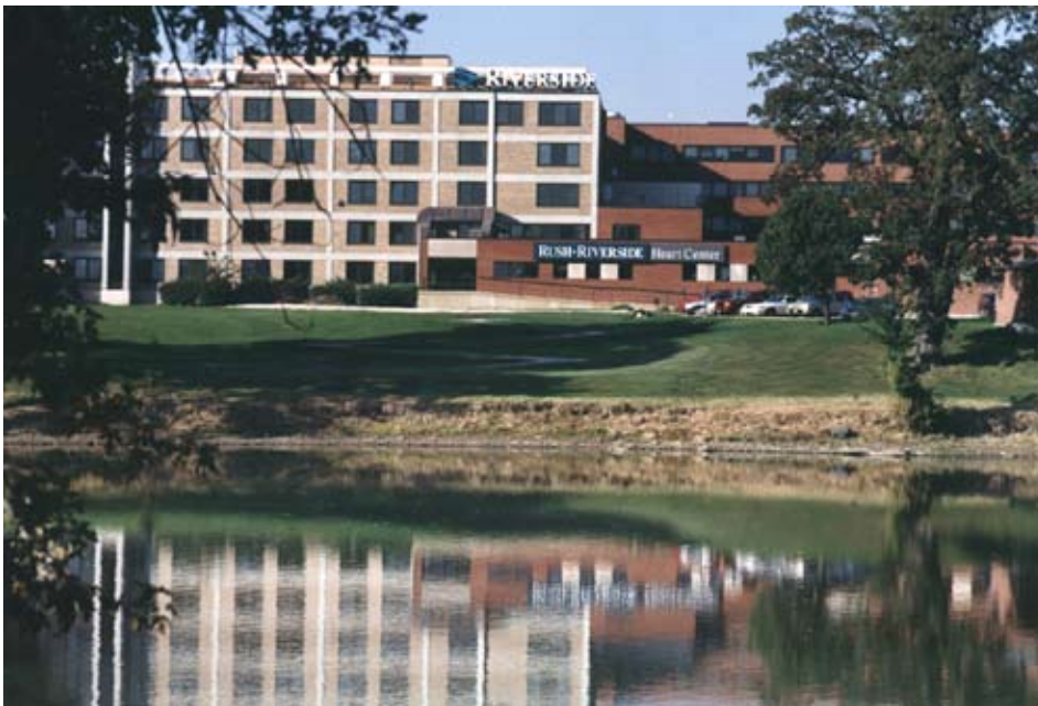
Riverside Medical Center, a 500,000 square foot facility, depends on H 2 Orange 2 117 for hydrogen peroxide cleaning efficiency.
